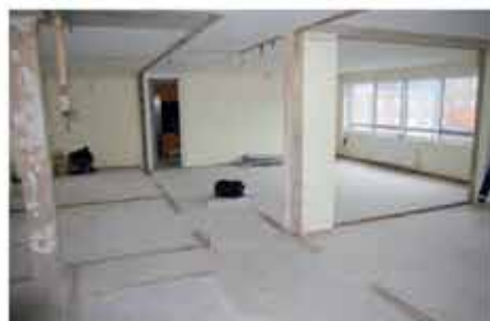
Figure 2: Shell after demolition of internal partitions
